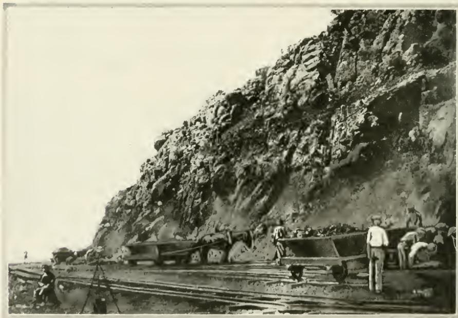
An ironstone quarry in the Iron Knob Mountain. Both the Iron Knob and the Iron Monarch mines are owned by the Broken Hill Company and the ore mined there is shipped by private railway to False Bay, then by steamer to Newcastle, where it is used in the Broken Hill Company's great steel plant.
