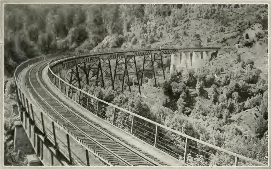
Viaducts of steel and concrete have replaced the wooden bridges on the main lines of the government railways. There are scores of them, because railroad building in New Zealand is a difficult task on account of the mountains and streams. Tunnels are frequent. One of them, now under construction on the South Island, will be five miles long.
